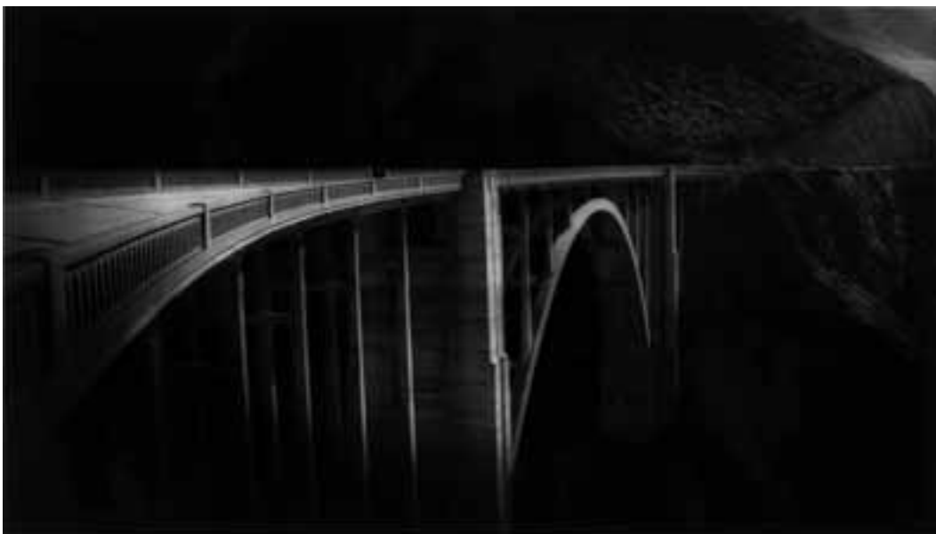
Bixby Creek Bridge, Big Sur, CA 1996 by Larry Wiese
